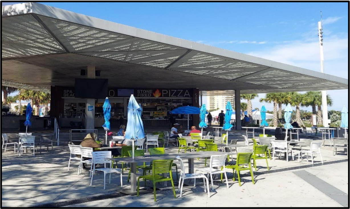
74. Shaded seating is provided at this café that overlooks the many activities, centrally located on the Pier plaza.
