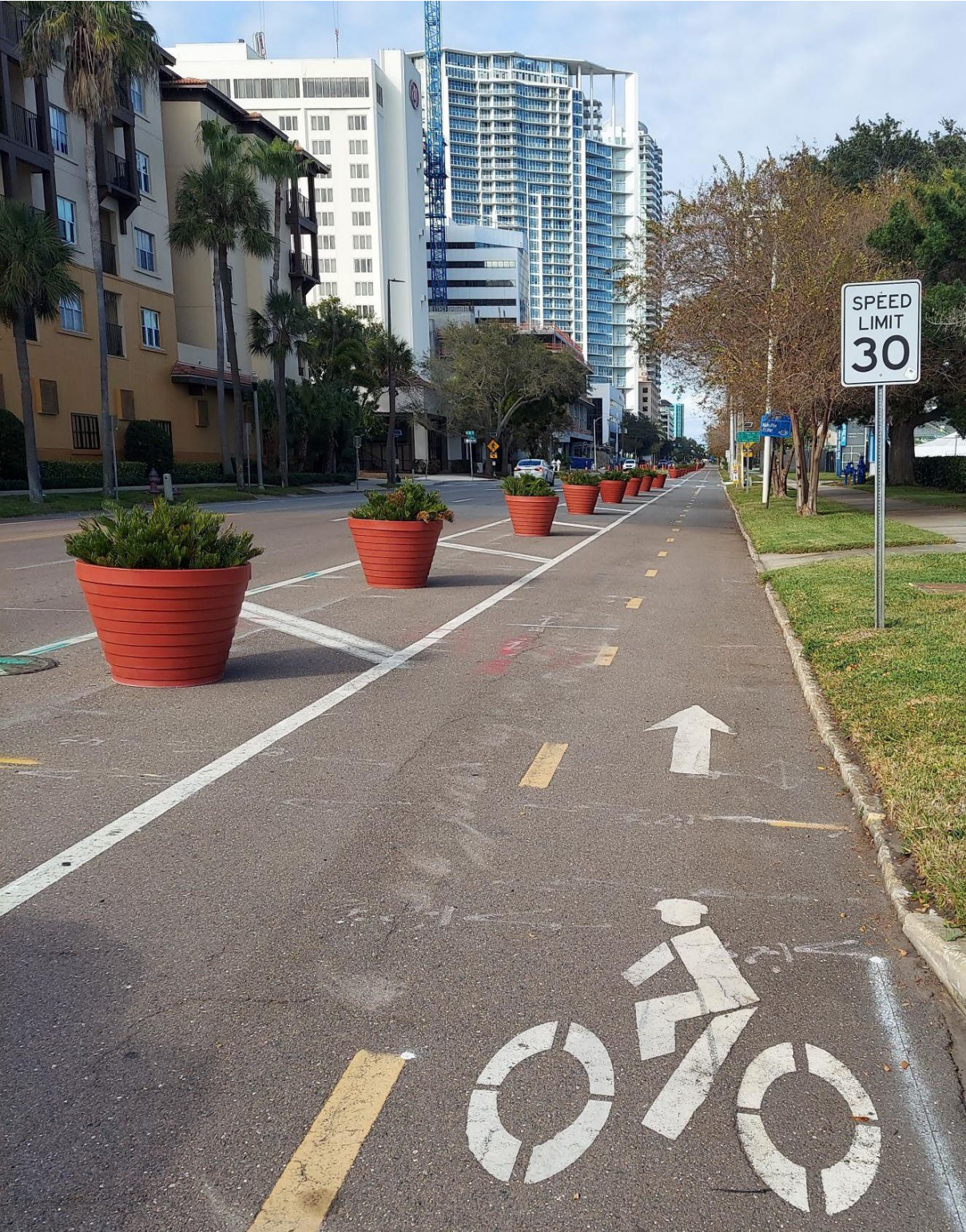
86. New bike lanes on 1 st Street S provide buffer area from vehicular traffic.
